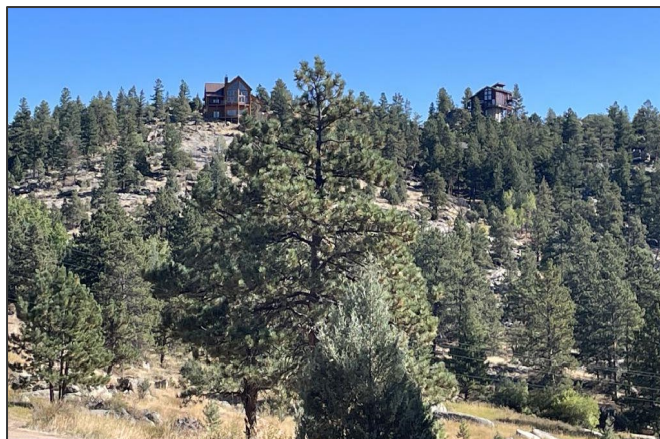
Homes built mid-slope and at the top of steep slopes and within ravines and draws are at greater risk of damage from wildfires. Dense vegetation near the structure exacerbates this risk. Photo credit: TEA.
